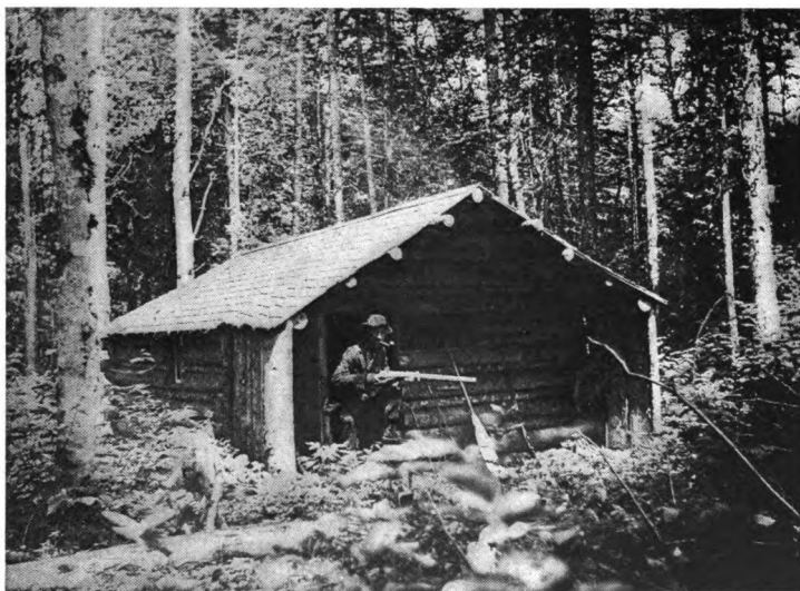
Mouse Tower. The Usual Type of Hunter's Cabin Does Not Always Make Provision for the Storage of Dry Firewood, which was the Chief Design of this Four Foot Projection.
