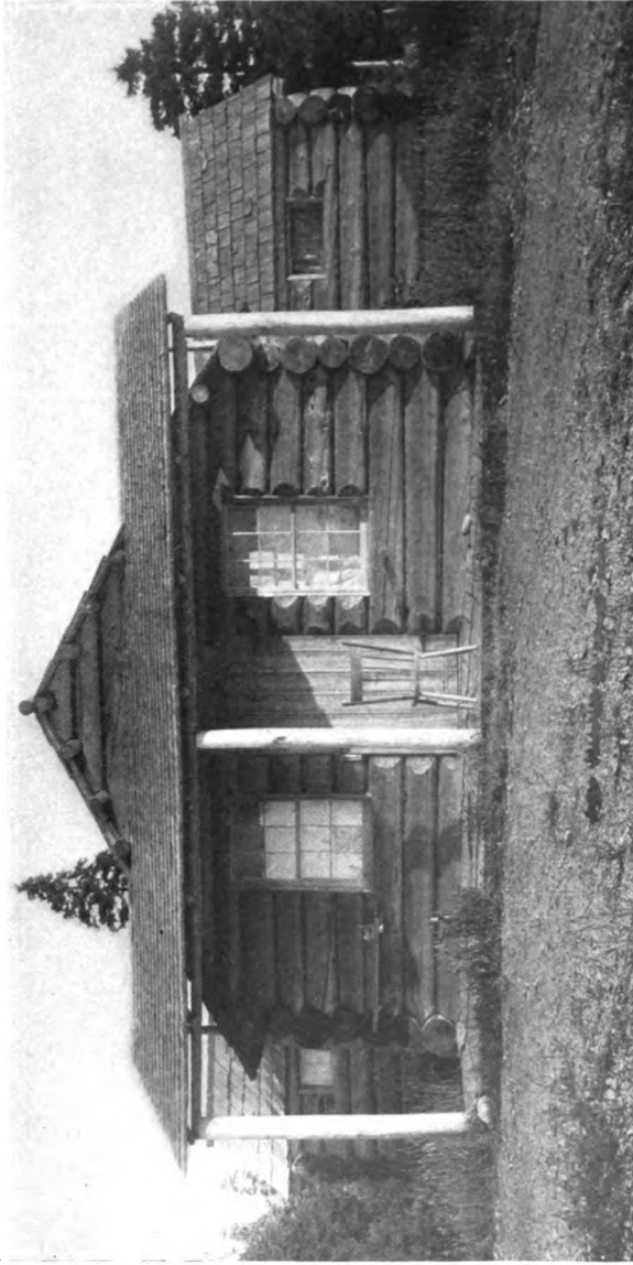
Note the Beveling of the Logs Around the Windows and Doors. Shows the Method of Setting in Rafters when Run Lengthwise of the Cabin.
